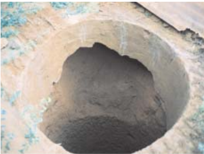
Pit collapse and cave-in, fueling perceptions of the dangers of latrines
