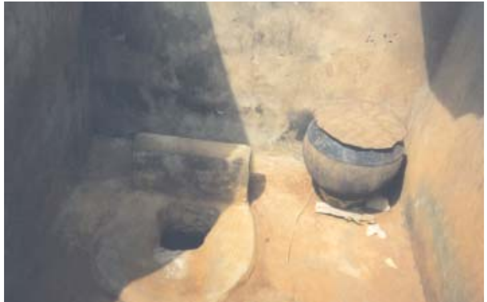
Customization and personalization of a latrine.
